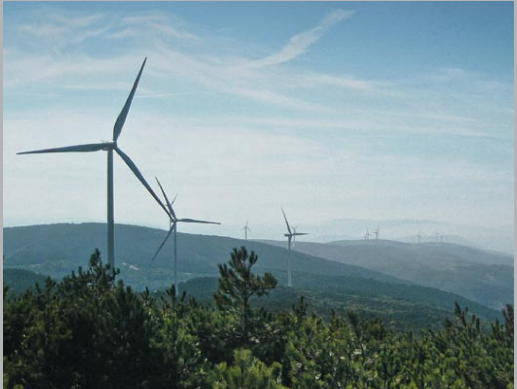
Bandirma wind farm, eastern Turkey
