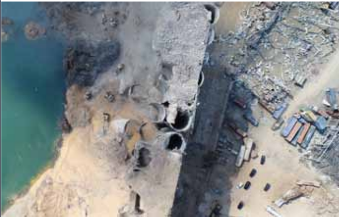
Inspection ▶ Humanitarian Aid ▶ Disaster response planning Beirut explosion - GSCF (Groupe de Secours Catastrophe Français), France
