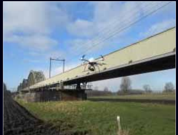
Railway bridge Inspection ▶ Maintenance Rijkswaterstaat, The Netherlands
