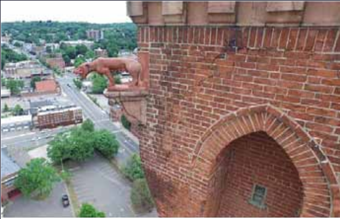
Inspection ▶ Heritage Sites & Historical monuments ▶ Erosion impact Industrial SkyWorks, Canada
