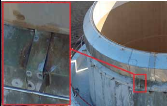
Inspection ► Maintenance ► Industrial sites ► Chimneys Force Technology, Denmark
