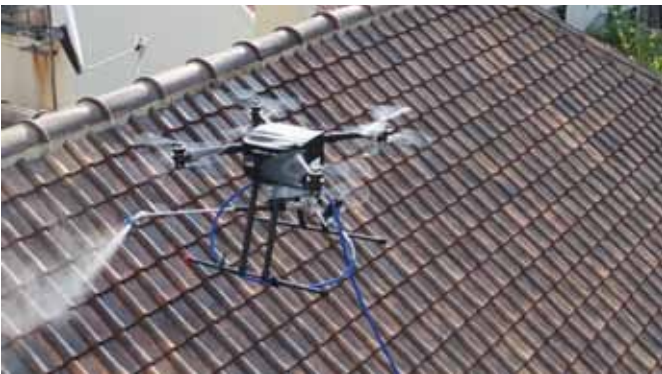
Roof Spraying (moss & lichen eradication) CleaningFly, France
