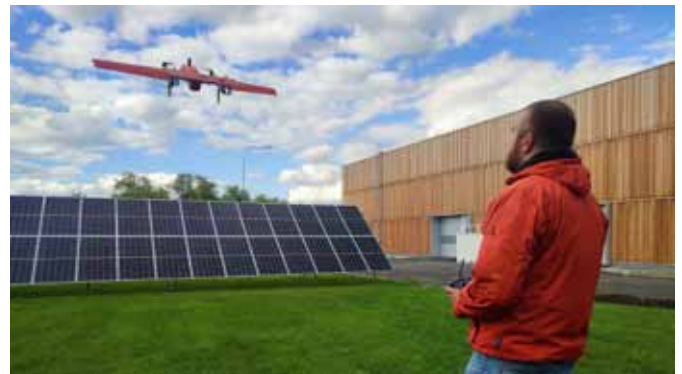
Solar Panel Inspection Fixar 007 - Fixar, Latvia
