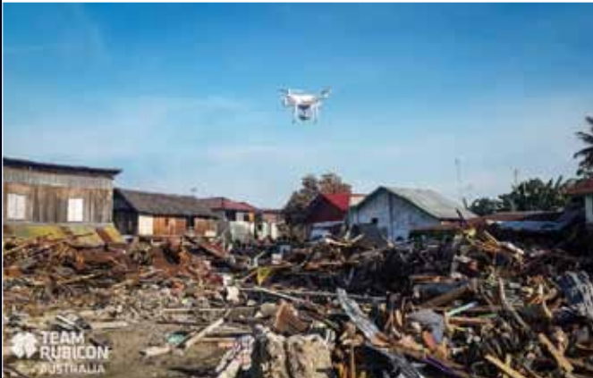
Inspection ► Public Services & Safety ► Post disaster - Natural (tsunami) Team Rubicon, Australia - for National Board For Disaster Mgt, Indonesia
