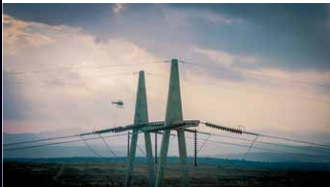
Powerline Inspection ▶ Maintenance Robot Aviation, Norway
