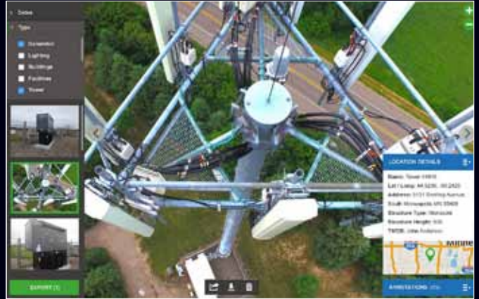
Inspection ► Maintenance ► Infrastructure ► Antennae Sentera, USA
