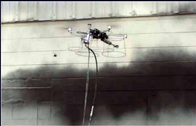
Spraying ► Construction ► Paint Spray Painting Drone (PoC) - Apellix, USA
