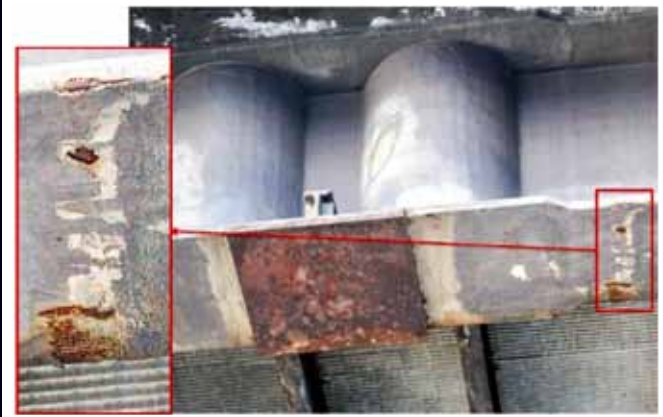
Inspection ► Mining & Exploration ► Offshore platform ► Corrosion Cyberhawk, UK
