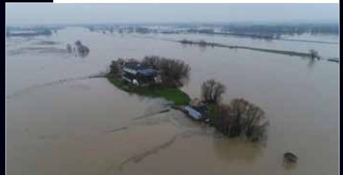
Post Flood Area Observation ▶ Public Services & Safety Rijkswaterstaat, The Netherlands
