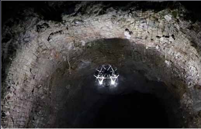
Inspection ► Mining & Exploration ► Mine tunnels Elios 2 - Flyability, Switzerland
