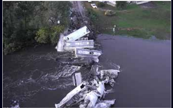
Inspection ▶ Insurance ▶ Post-accident/disaster ▶ Bridge collapse Aftermath of Iowa Rail Bridge Collapse - Sioux County Sheriff, USA
