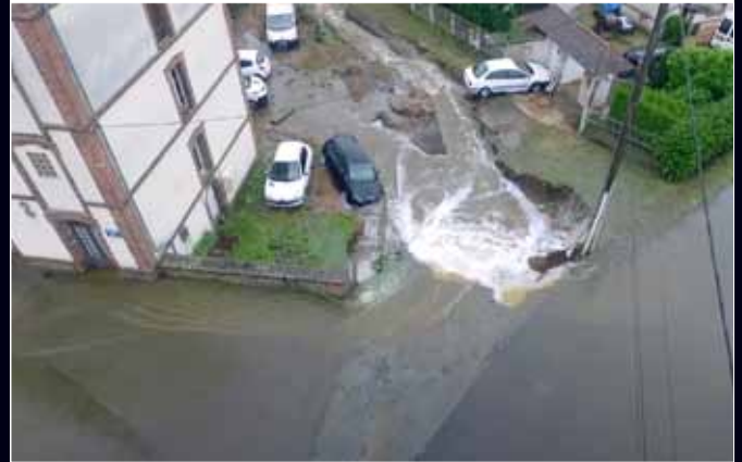
Inspection ▶ Insurance ▶ Meteorological damage impact evaluation on: Infrastructure Drone Malin, France
