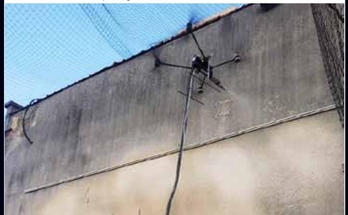
Spraying ► Construction ► Mortar coatings
